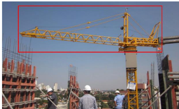
Figure 1: An example of bounding box that detect the boom of a tower crane
