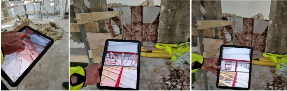
FIG. 7: Filtering BIM objects during a renovation project to understand which should be demolished and which should be kept (Case project: SB47).
