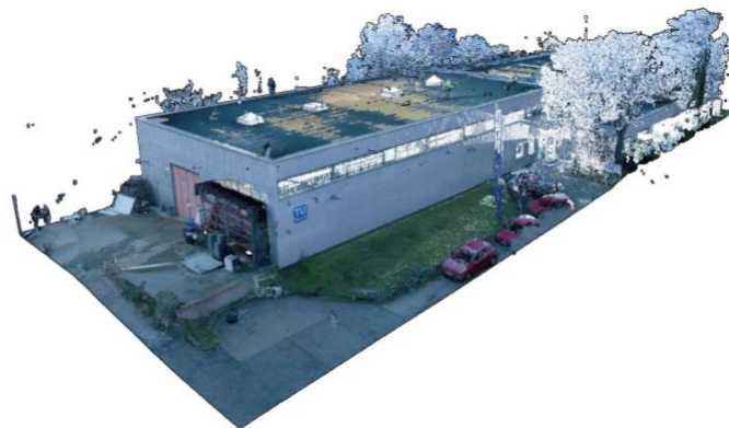
FIG 6: Point Cloud 1 from laser scan of the use case, as generated by company 1
