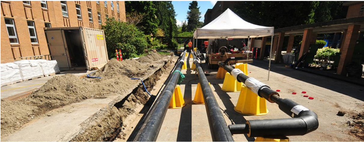
FIG. 4: Pipe installation for UBC's Academic District Energy System (ADES).
