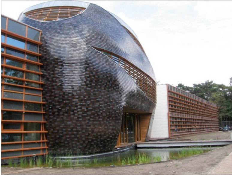
FIG.4: The new headquarters of the World Wildlife Fund in Zeist, The Netherlands, is claimed to be CO 2 neutral. It is based on the skeleton of an existing office building and is largely built from reused materials.
