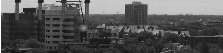
FIG. 7: UM Central/Medical campus School of Public Health construction site identified as highest point
