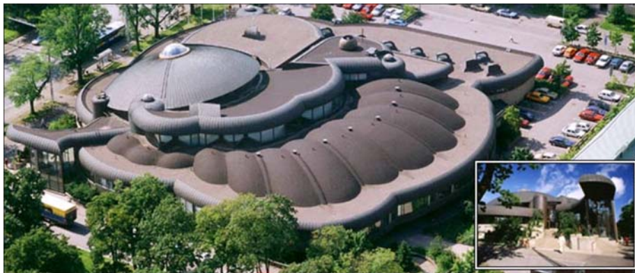
FIG. 6: Tampere city library Metso by Reima Pietilä 1986 is strongly emphasized by the curved concrete beams and concrete elements in the roof structure. Metso ( capercaillie , lat. Tetrao urogallus ) which is a largish bird living deep in the forests, has given the shape to Pietilä's library.
