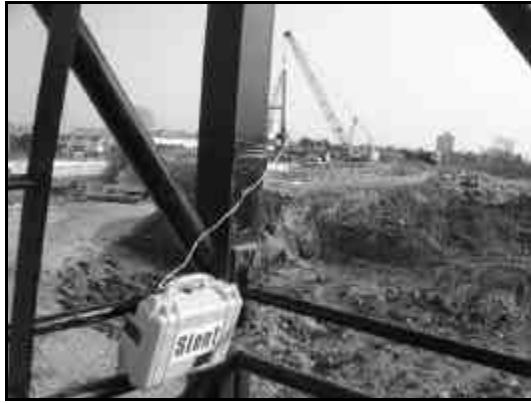
FIG.7: Tower crane mounted WNC.
