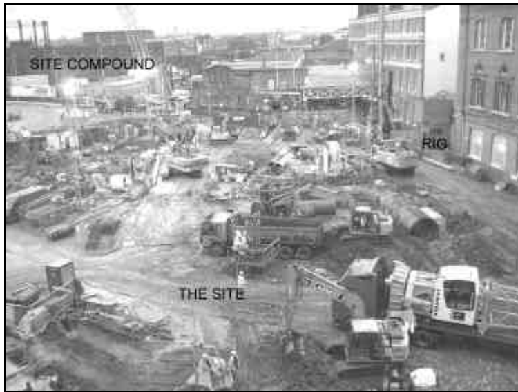
FIG.3: Kings Cross construction site showing location of site compound
